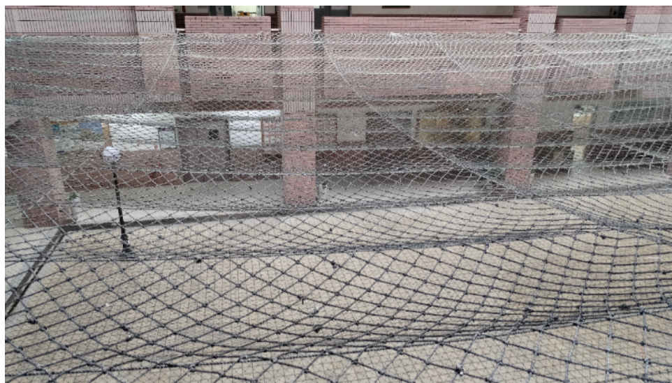
A safety net situated at the center of the building
